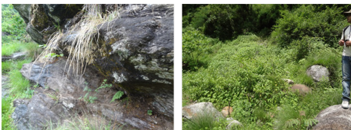
Fig. 3: Augen gneiss (left side, observed near the surge tank) and big boulders of gneiss and schist (right side, observed near the proposed powerhouse area).
