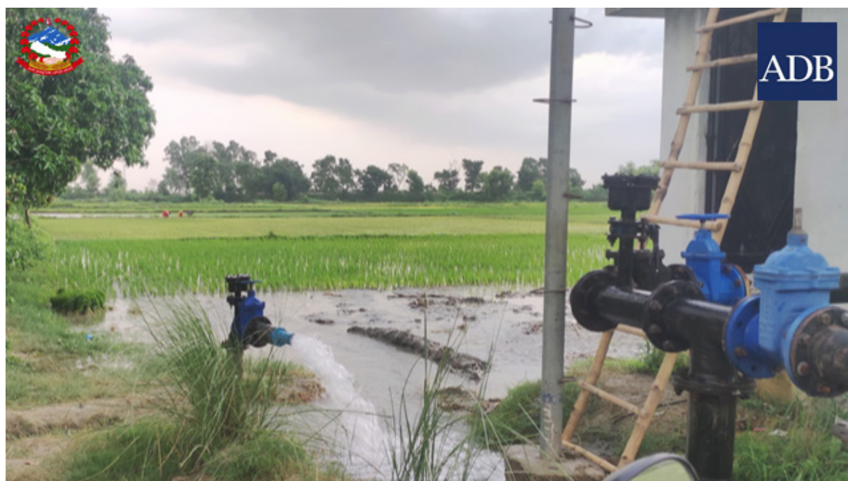
Fig. 2: Pilot project constructed in Paroha, Rautahat (Photo source: DWRI and ADB).
